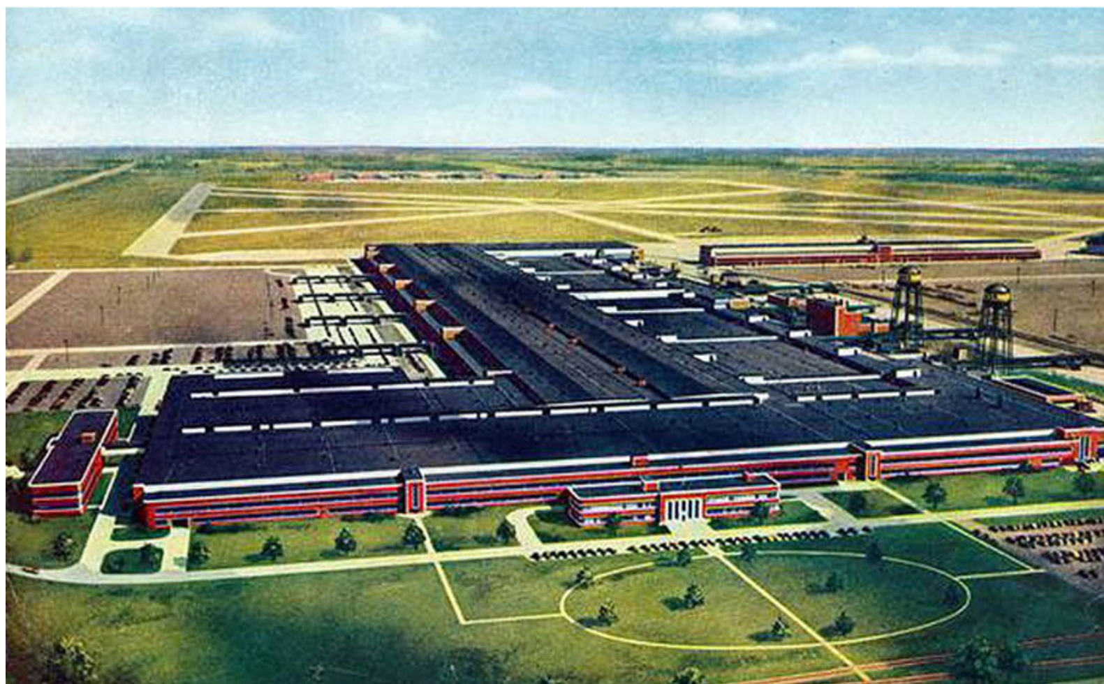
Willow Run, Michigan: An air view of progress in the Ford Motor Company's construction of a vast bomber plant.
