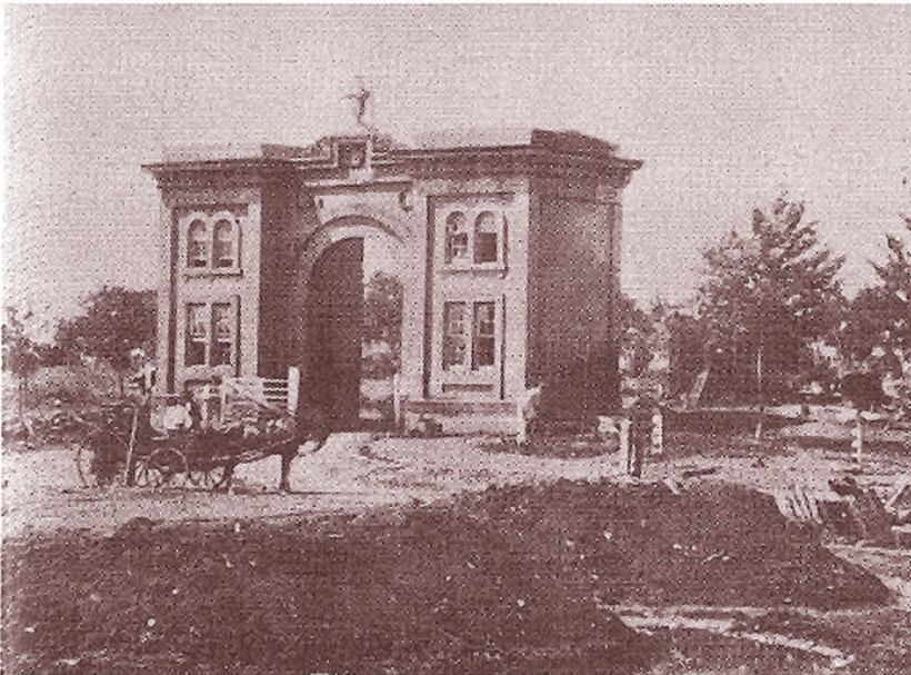
Lunettes, or artillery defense works, on the crest of East Cemetery Hill. The entrance gateway to the public cemetery, which is still in use, appears in the background on the Baltimore Pike. Brady photograph.
