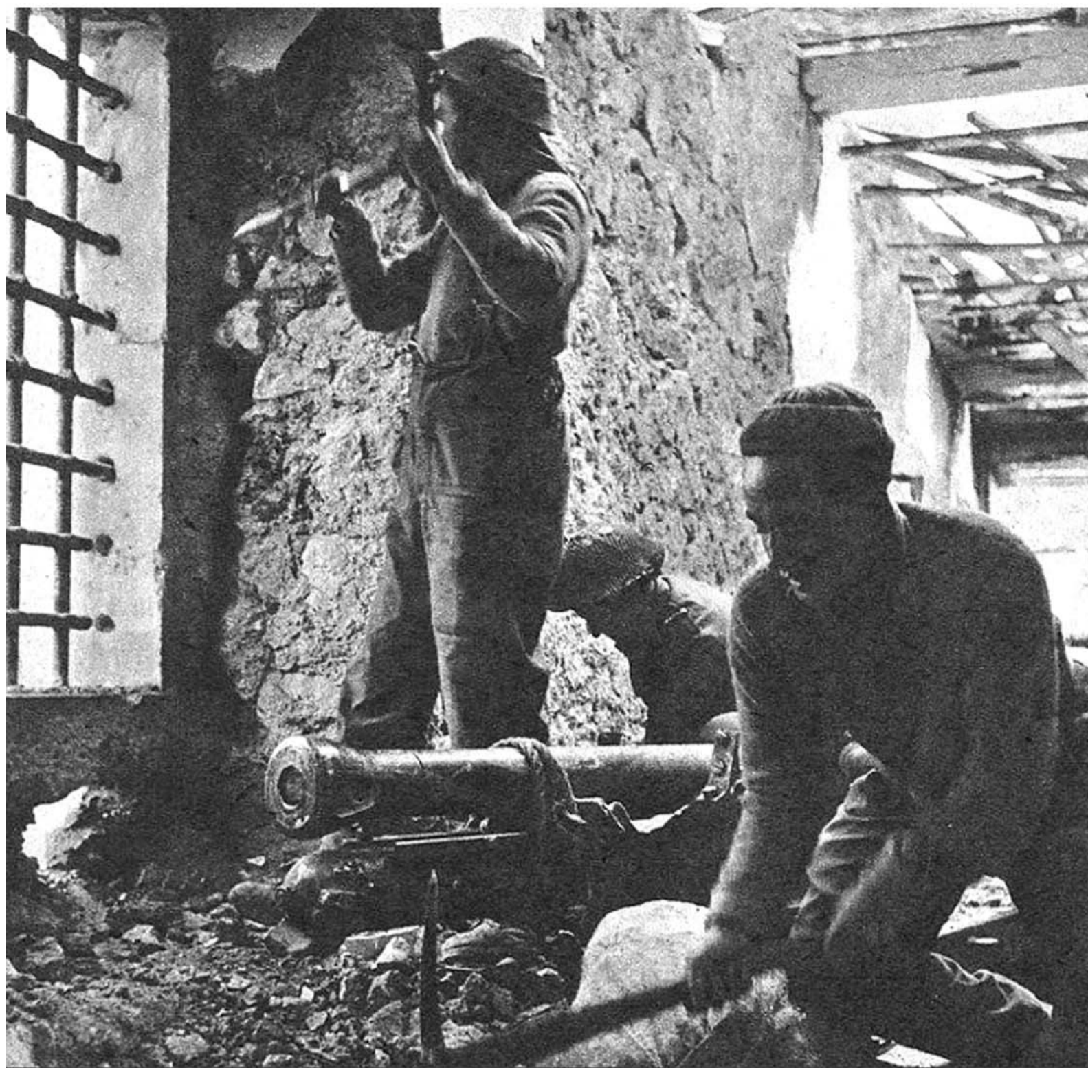
IN A HOUSE WHERE WALLS ARE SO THICK THAT IT IS A FORTRESS, NEW ZEALANDERS INSTALL ANTITANK GUN.
