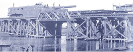
Trestles had to be strengthened to carry the immense weight—275 tons each—of the gun cars as they left St. Nazaire for the front.
