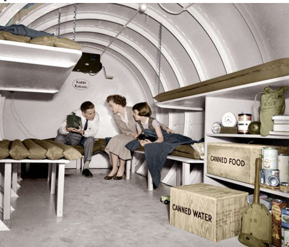
Manufactured by Walter Kidde Nuclear Labs, the Kokoon has its own gasoline generator, toilet, filter.
