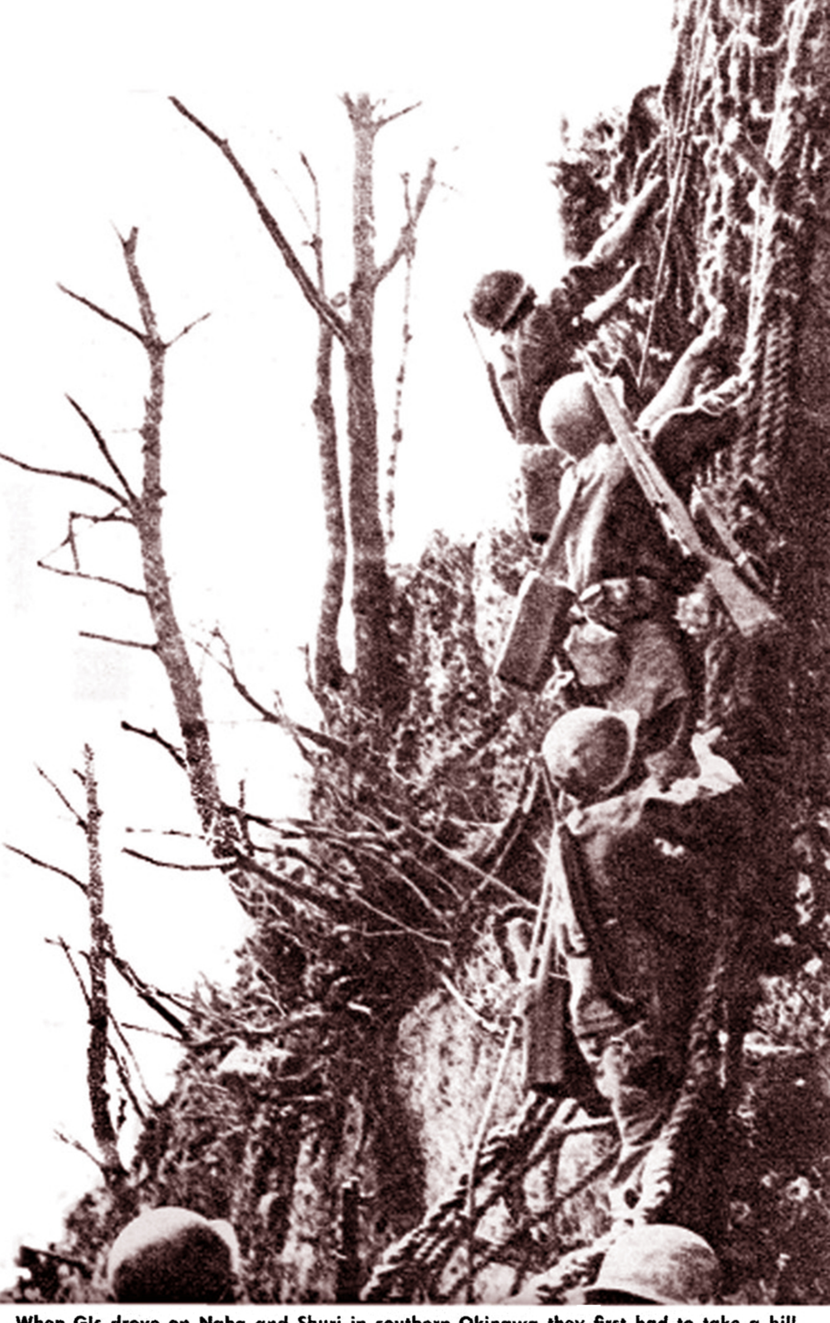
When GIs drove on Naha and Shuri in southern Okinawa they first had to take a hill known as the "Escarpment," a network of caves and pillboxes covering the approaches to the two cities. Here men of a combat-engineer outfit carry satchel charges up the "Escarpment" to blow out Jap cave entrances. They use ships' cargo nets to scale it.
