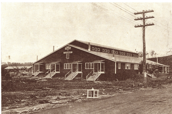
Y. M. C. A. AUDITORIUM AT CAMP DEVENS, AYER, MASS.
