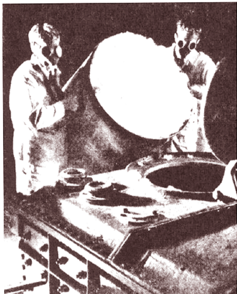
Cotton-linters are dumped into mixer with chemicals to form cellulose solution
