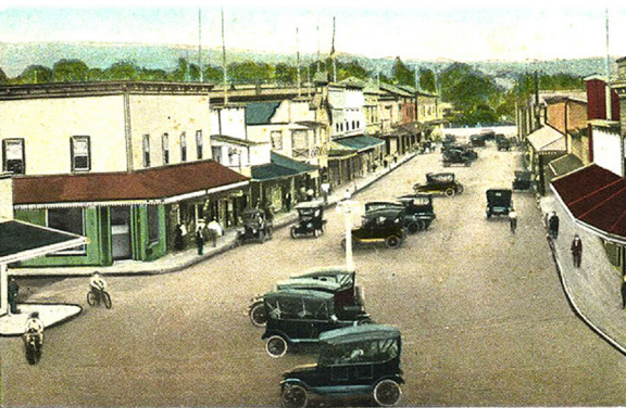
KAMEHAMEHA AVENUE, HILO, HAWAII.
