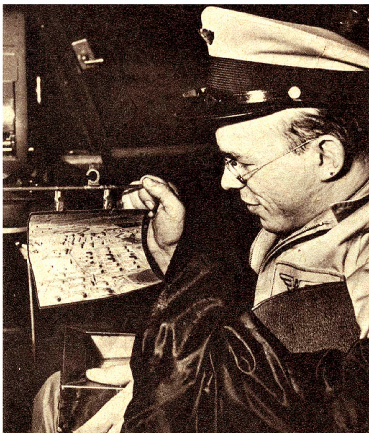
The development of the paper negative, used instead of film for speed, is done in less than a minute with the aid of a lightproof black bag and specially built developing and fixing tanks.
