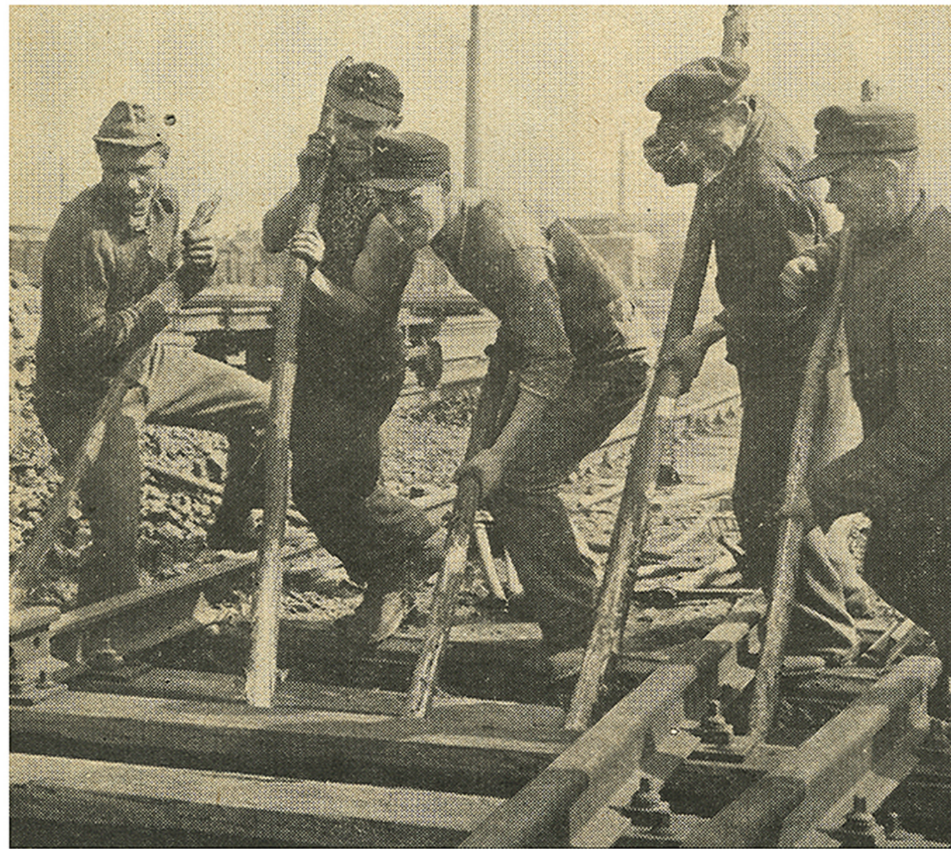
Heave-Ho. German workers repair rails,
