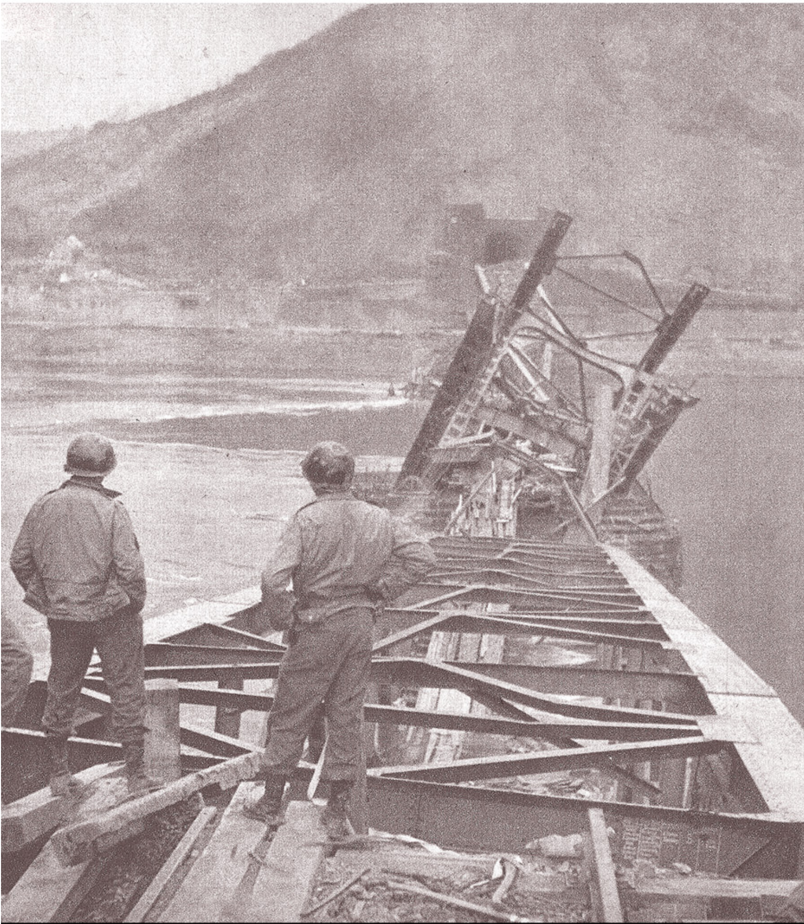
But after its 10 brief days of glory, there was nothing left of the bridge at Remagen but these broken beams and a few odd planks floating lazily down the Rhine.
