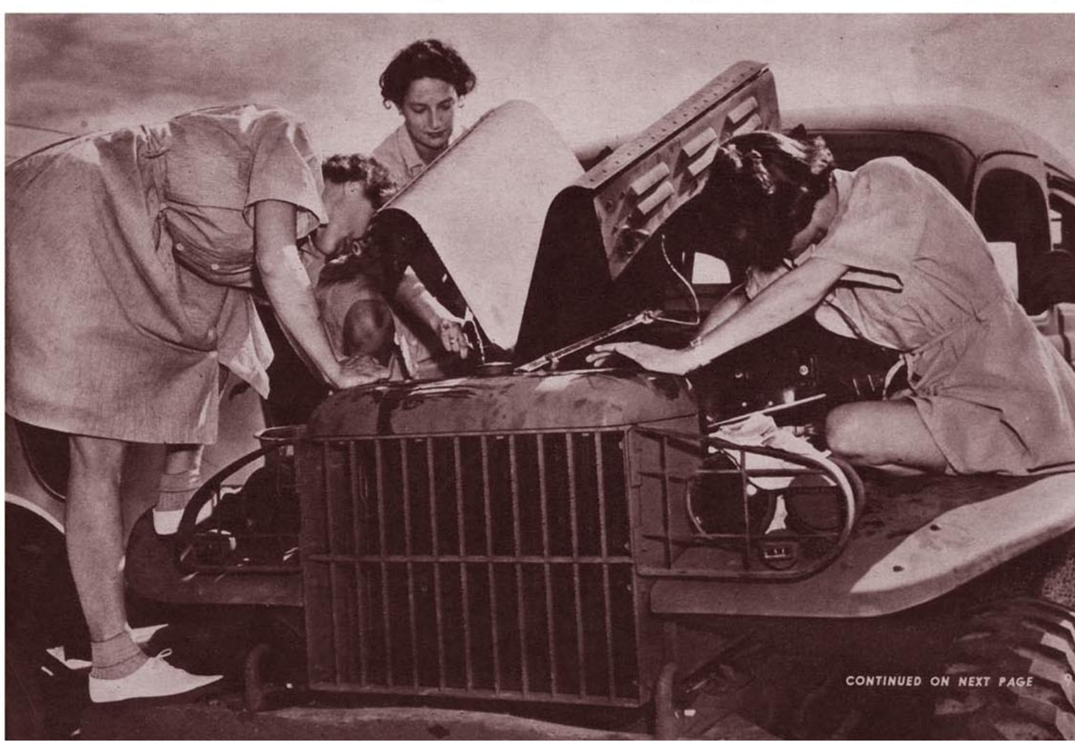
TAUGHT MOTOR REPAIR AND MAINTENANCE IN A SPECIALIZED CORPS FOR AUXILIARIES, THESE GIRLS WASH ENGINES WITH KEROSENE PRIOR TO INSPECTION
