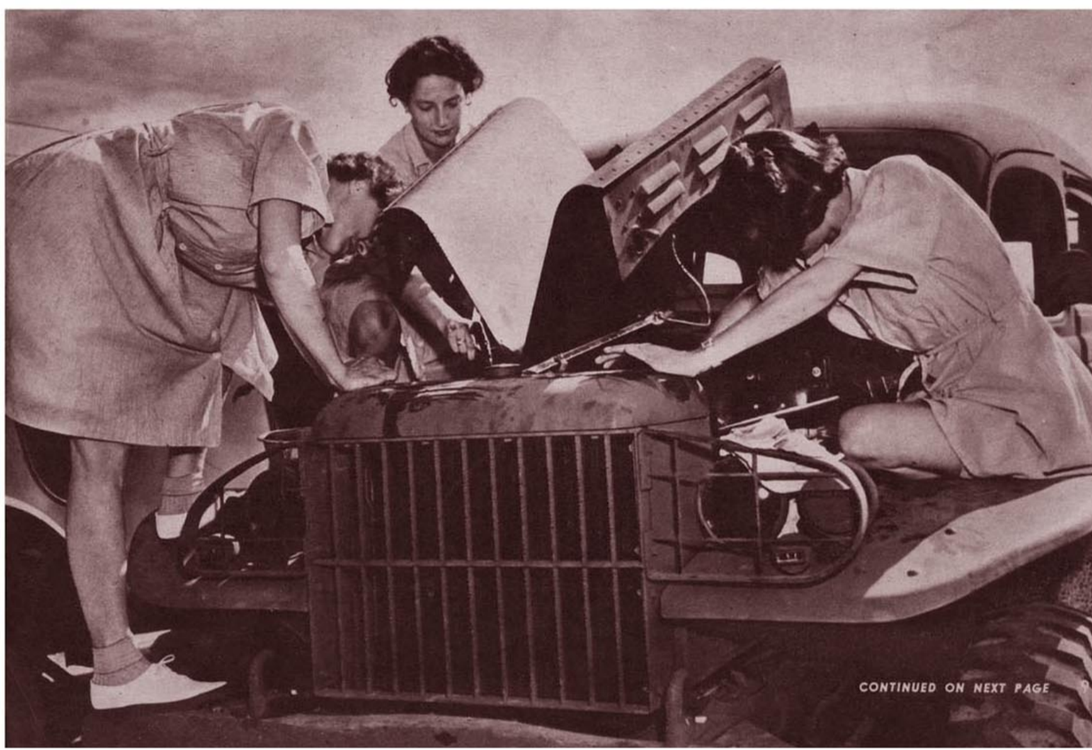
TAUGHT MOTOR REPAIR AND MAINTENANCE IN A SPECIALIZED CORPS FOR AUXILIARIES, THESE GIRLS WASH ENGINES WITH KEROSENE PRIOR TO INSPECTION
