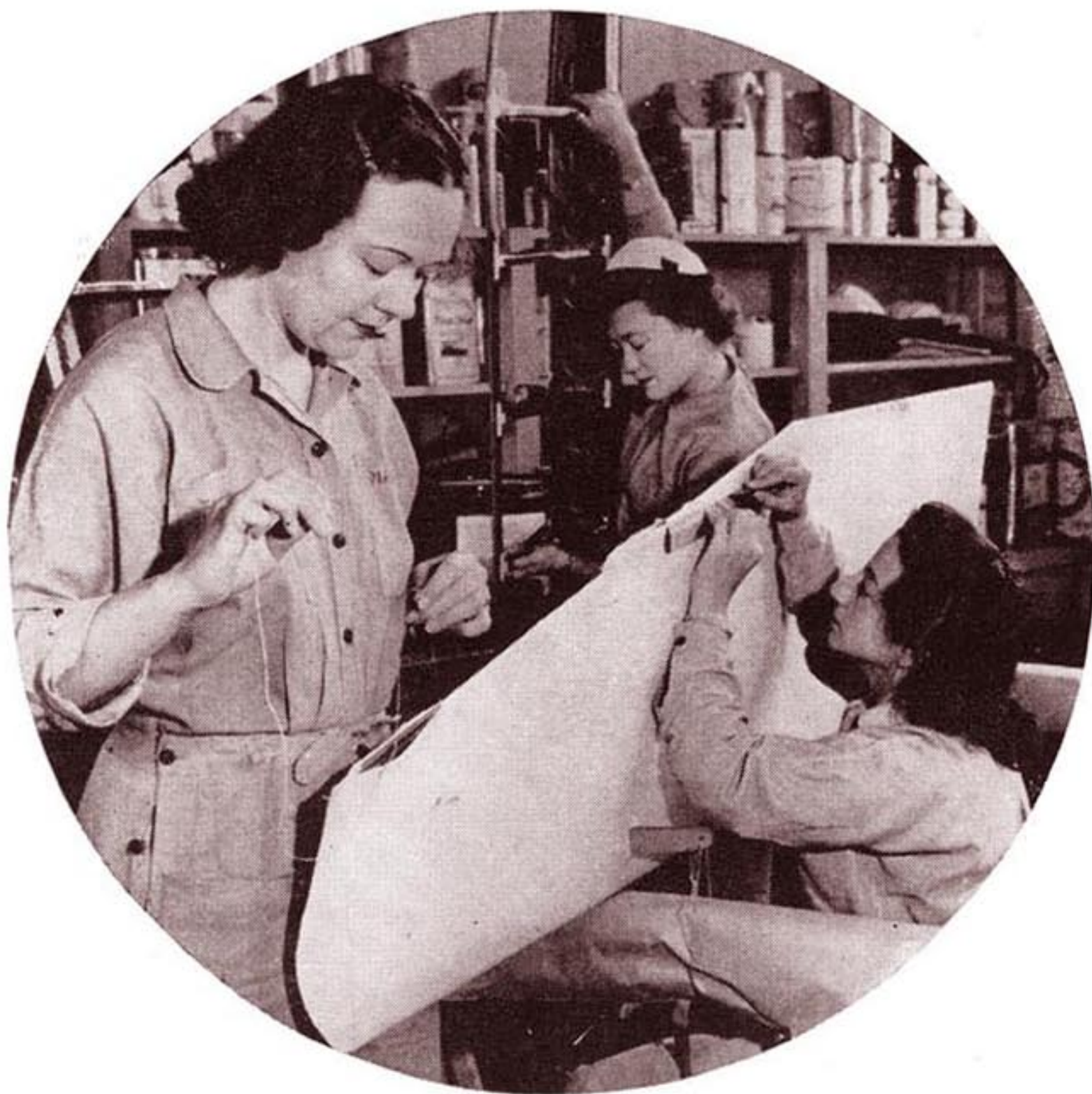
Above: SPARS are veteran plane fabric repairers at Coast Guard's San Diego air station, making damaged plane wings usable again.
