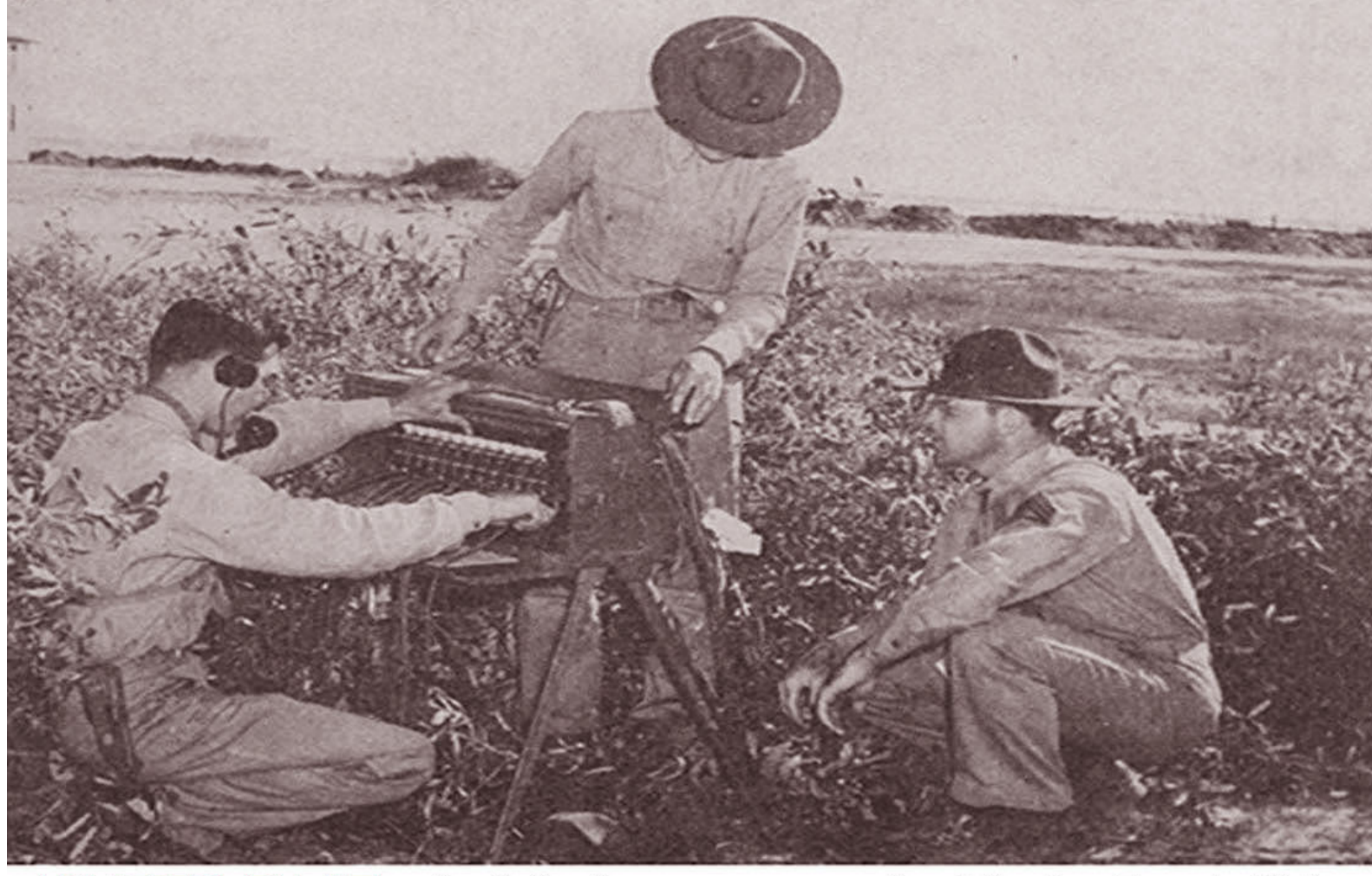
AT THE BASE: At left, instructors at the Marine Base's Telephone School are setting up an emergency telephone system for a demonstration. This school's course is an intensive one. Good communications set up by Telephone School graduates have been very important in the Solomons Islands campaign.
