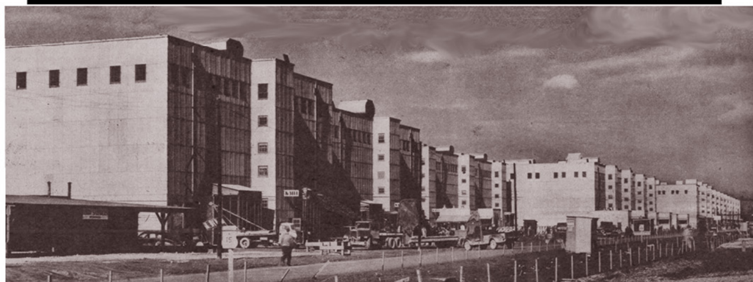
One of the giant production plants of the Clinton Engineering works at Oak Ridge, Tennessee.
