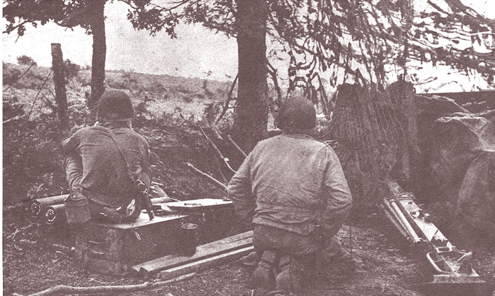
Tarp covers tank destroyer's 57-mm gun to protect it from light rain. Enemy are in clearing 100 yards ahead.
