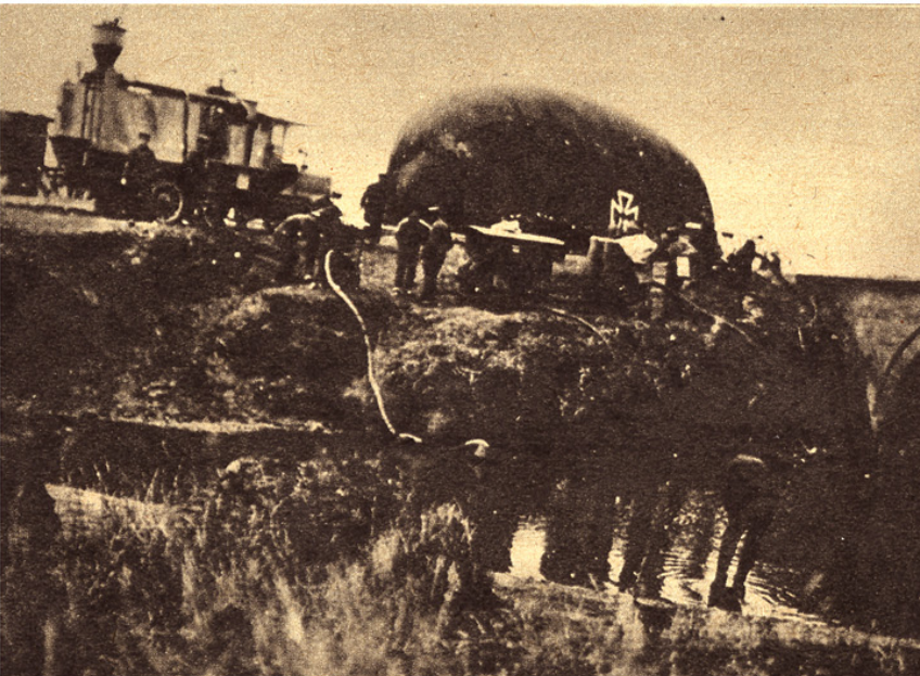
THESE TENTS, covering a gas-filled balloon, caved in from snow.
