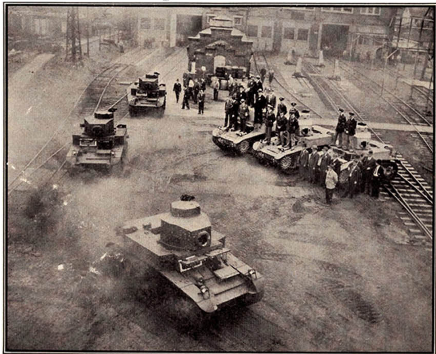
... as ACF rolls light tanks off the line at Berwick, Pa.
