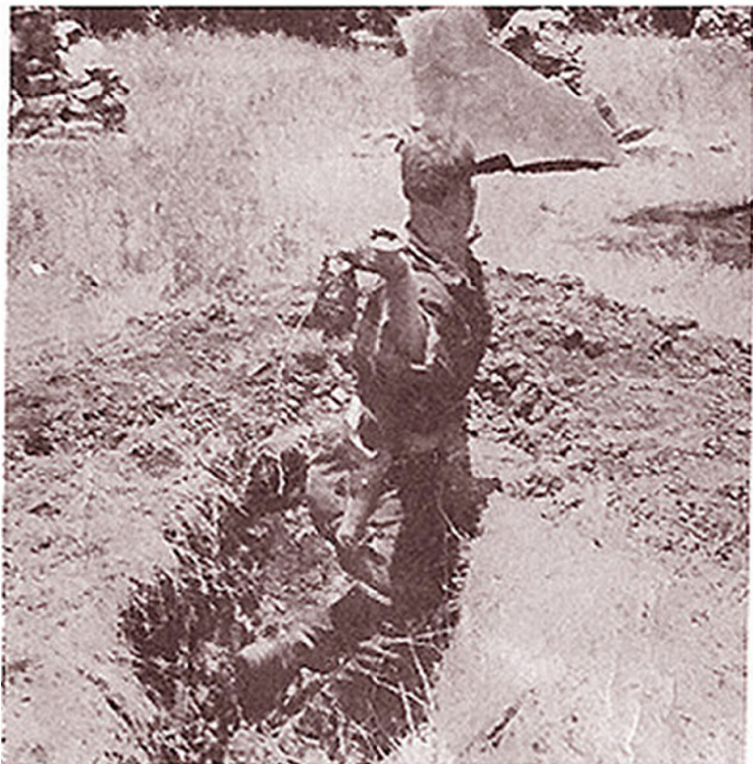
ABOVE: From a slit trench, this TD soldier hurls a "sticky grenade" at an upright piece of concrete representing a tank.
