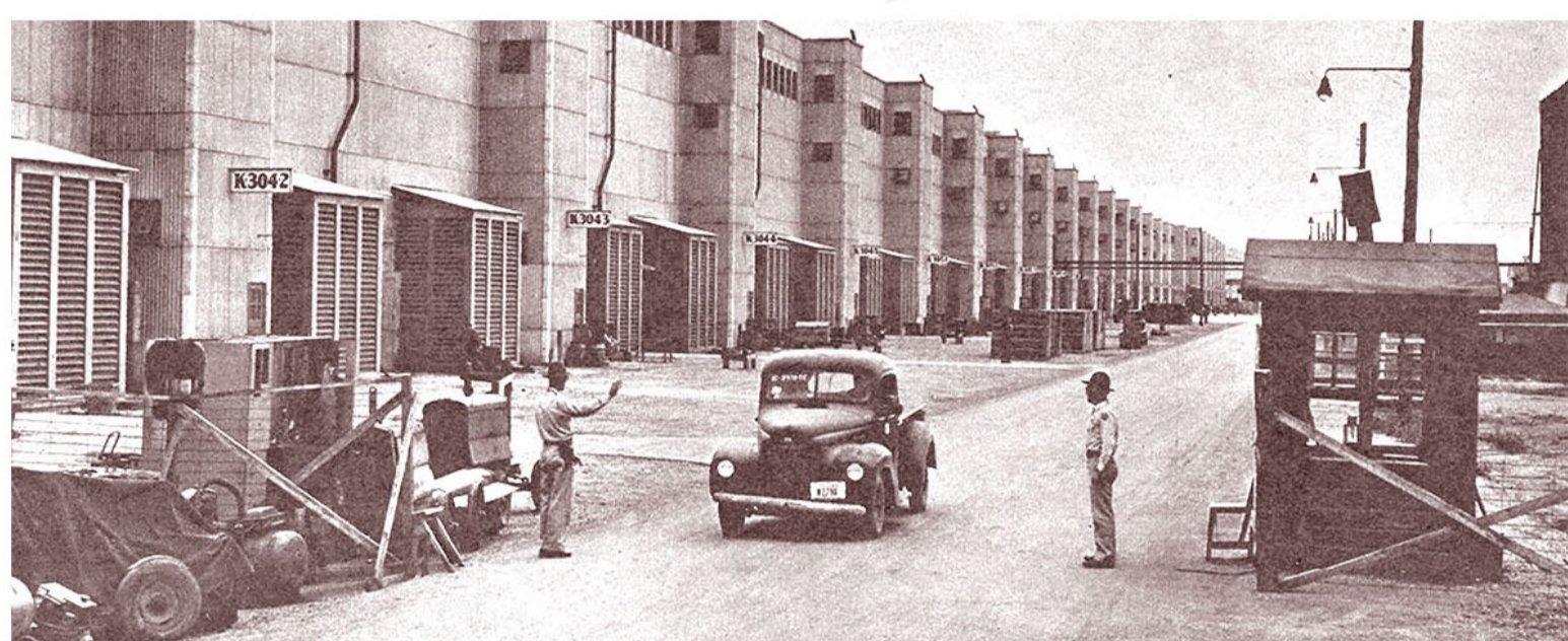
Guards stop cars or trucks coming in or out of the Carbide & Carbon Chemicals Corp. plant.
