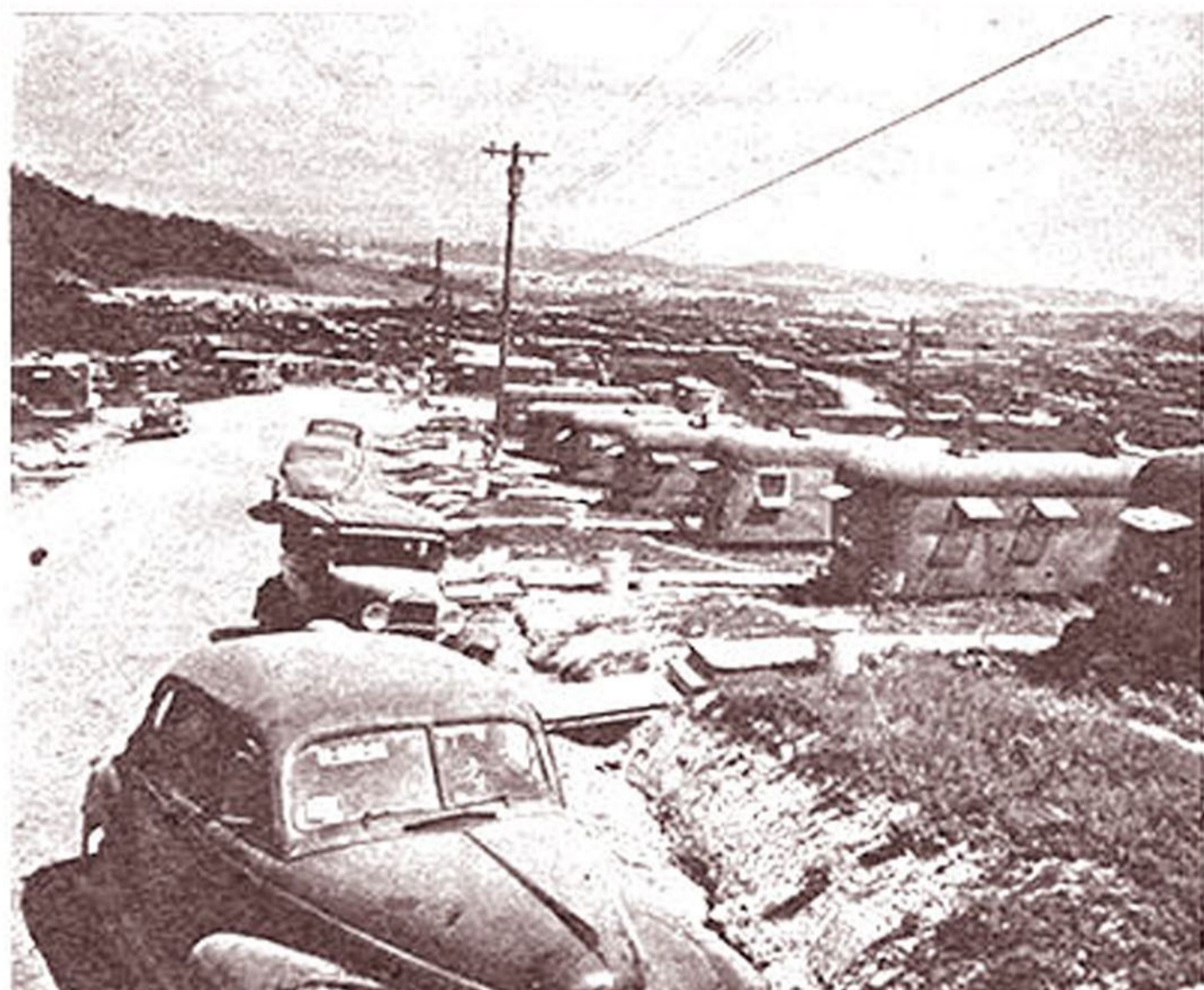
Hundreds of plant workers live in trailers like this one, but most GIs are quartered in barracks.
