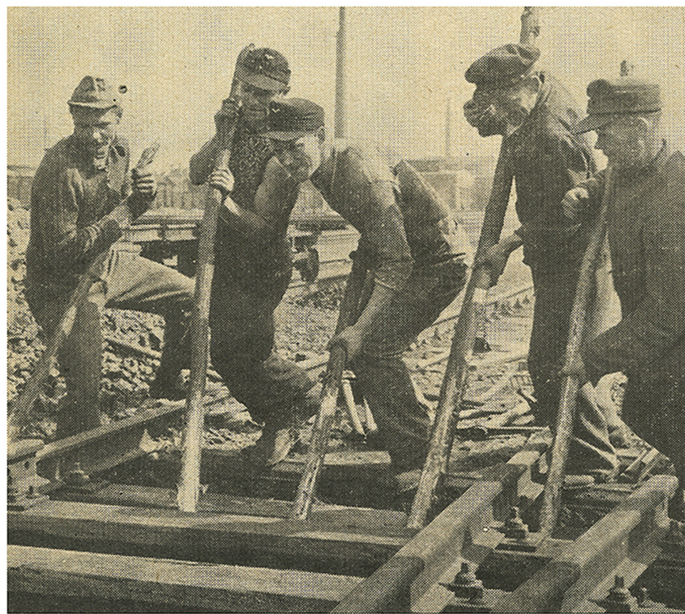
Heave-Ho. German workers repair rails,
