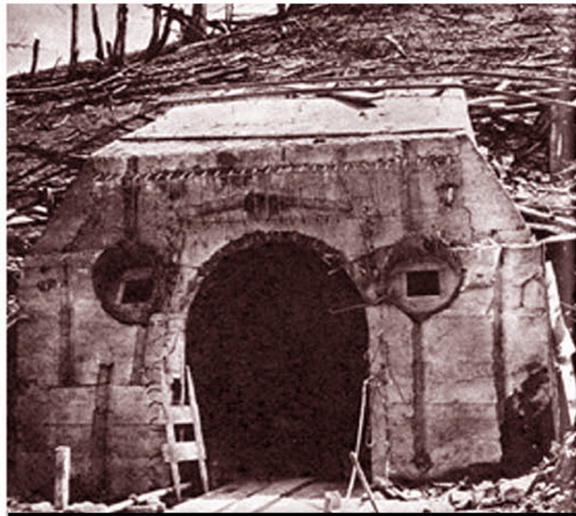
Entrance to luxuriously furnished tunnels under the Berghof .
