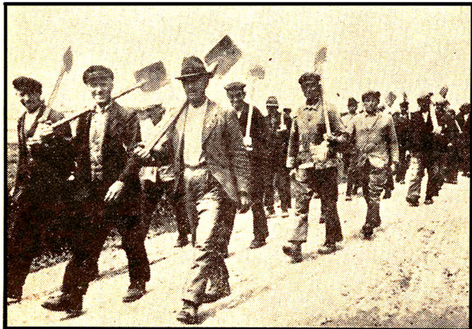
Last act in Germany: Workers march out to build fortifications
