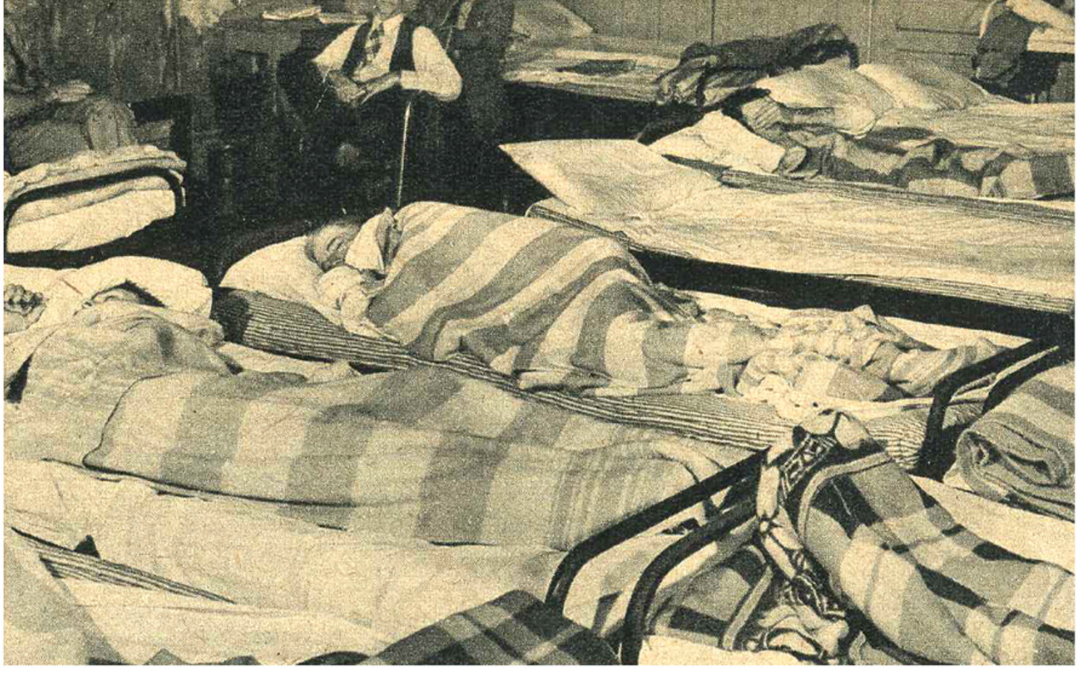
CONSTRUCTION WORKERS in Alexandria, La., had to be satisfied with sleeping quarters such as this 37-bed dormitory. At times they slept in shifts. To make matters worse, some of men housed here had influenza.
