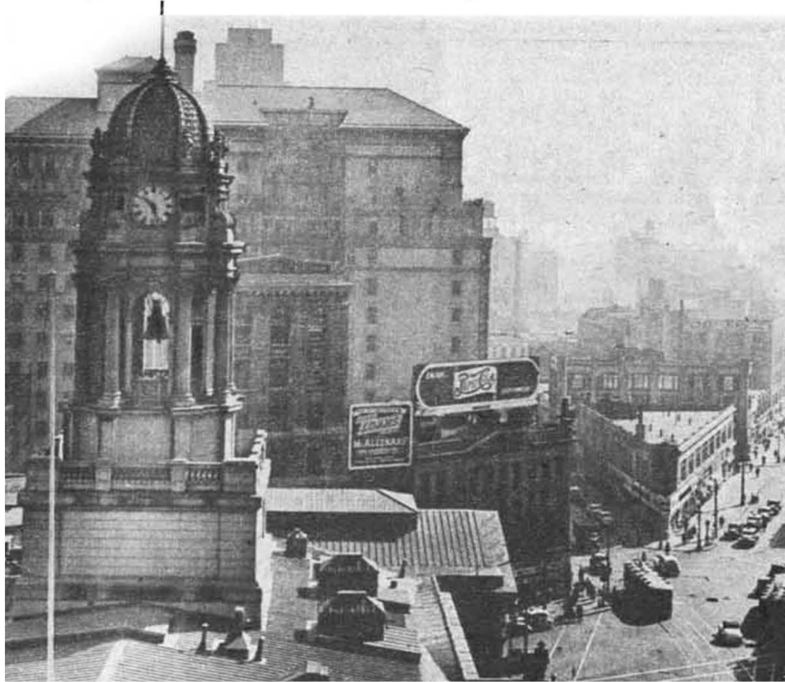
Borough Hall looks the same. But people can't get used to Fulton Street naked without it's El.
