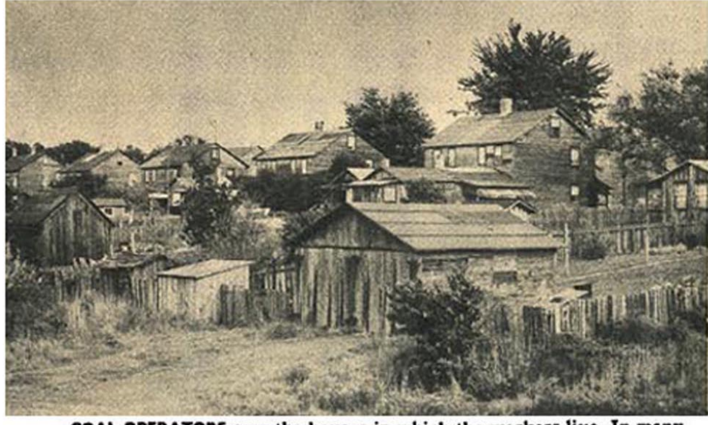
COAL OPERATORS own the houses in which the workers live. In many areas these are the only homes and the rents are unjustifiably high.
